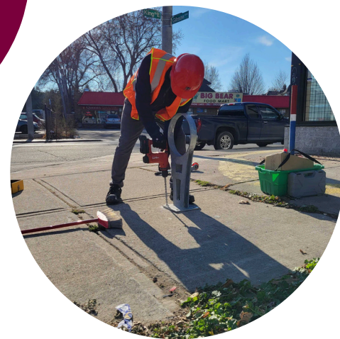
Installing a hammer hoop bike rack at a Shelter Health Network located in downtown Hamilton. Photo Credit: Alison Carlyle, City of Hamilton
